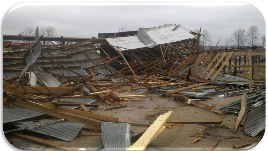
Figure 9: Tornado damage from storm on 2/28/2011.
